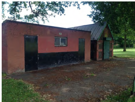
Disused building at Longlands Recreation Ground.
